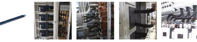
IBSB is the ideal ready-to-install flexible wire replacement solution that is specifically designed for connections to all molded case circuit breakers, including the most compact breakers on the market. It connects to the front access terminals of the breakers without any additional accessories, such as angular connectors, spreaders, ring terminal connectors or extenders. IBSB is available in cross section of 25 to 240 mm<sup>2</sup> (49.34 to 273.65 kcmil), lengths from 165 to 1,130 mm.
