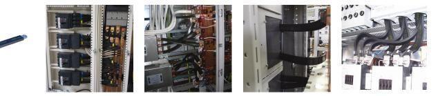
IBSB is the ideal ready-to-install flexible wire replacement solution that is specifically designed for connections to all molded case circuit breakers, including the most compact breakers on the market. It connects to the front access terminals of the breakers without any additional accessories, such as angular connectors, spreaders, ring terminal connectors or extenders. IBSB is available in cross section of 25 to 240 mm<sup>2</sup> (49.34 to 273.65 kcmil), lengths from 165 to 1,130 mm.
