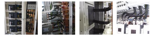
IBSB is the ideal ready-to-install flexible wire replacement solution that is specifically designed for connections to all molded case circuit breakers, including the most compact breakers on the market. It connects to the front access terminals of the breakers without any additional accessories, such as angular connectors, spreaders, ring terminal connectors or extenders. IBSB is available in cross section of 25 to 240 mm<sup>2</sup>, lengths from 165 to 1,130 mm.
