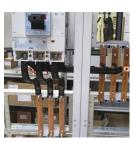
IBS Flat Insulated Braided Conductors are the ideal ready-to-install flexible wire replacement solution. They connect directly to the front access terminals of an electrical device without the need for additional accessories, such as angular connectors, spreaders, ring terminal connectors or extenders. IBS Flat Insulated Braided Conductors are available in cross section of 25 and 50 mm $^2$  (49.34 and 98.68 kcmil), lengths from 1650 to 1,130 mm, and amperages ranging from 177 to 274 A.
