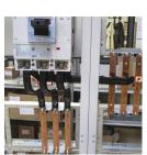
IBS Flat Insulated Braided Conductors are the ideal ready-to-install flexible wire replacement solution. They connect directly to the front access terminals of an electrical device without the need for additional accessories, such as angular connectors, spreaders, ring terminal connectors or extenders. IBS Flat Insulated Braided Conductors are available in cross section of 25 and 50 mm<sup>2</sup> (49.34 and 98.68 kcmil), lengths from 1650 to 1,130 mm, and amperages ranging from 177 to 274 A.
